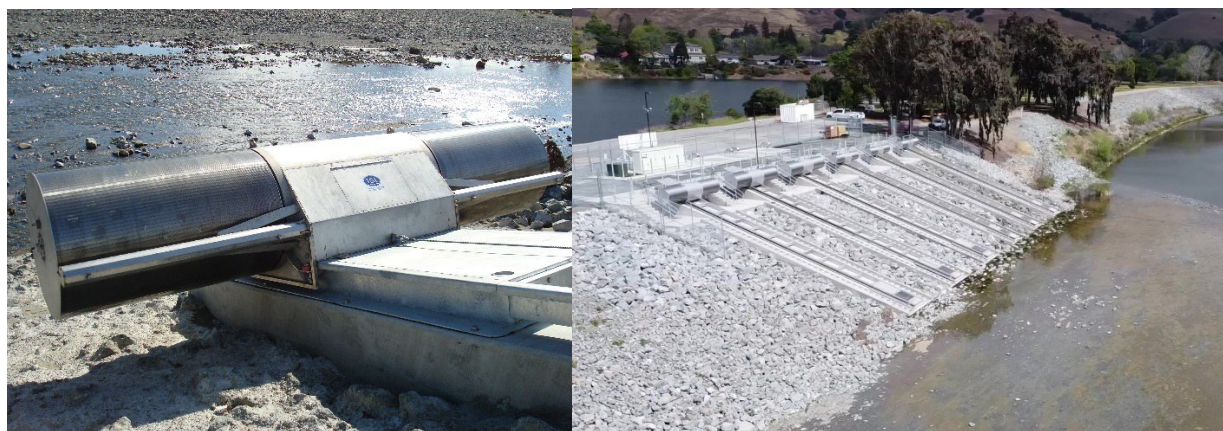
Figure 5-1: Single Shinn fish screen close-up (left), and the set of screens lined up on the northern bank of Alameda Creek (right).
